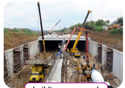
building a new road
